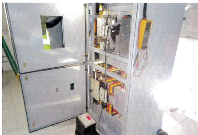
ACB TRIP UNIT TEST
