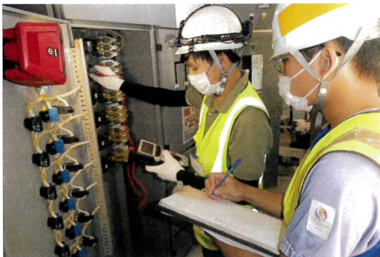
INSULATION RESISTANCE MEASUREMENT
