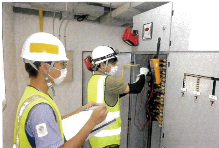
CAPACITANCE MEASUREMENT
