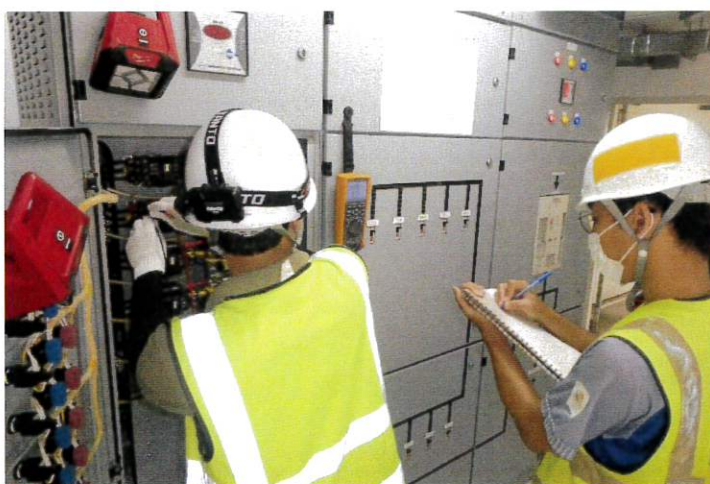
CONTACT RESISTANCE TEST
