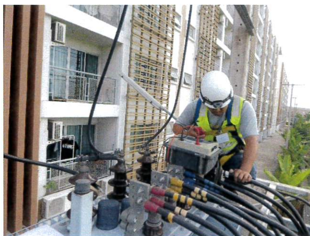
INSULATION RESISTANCE TEST
